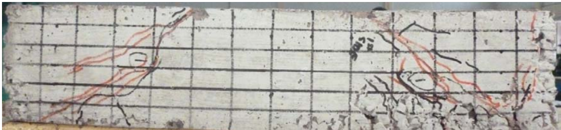
Figure-8. Crack patterns of specimens.
