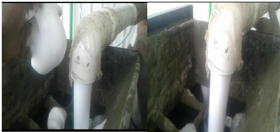
Figure-3. (a) & (b) Foam from outlet valve to a concrete mixer.
