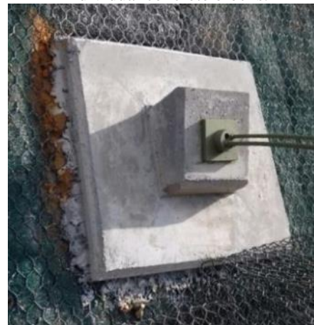
d) Individual concrete blocks with single twist mesh
