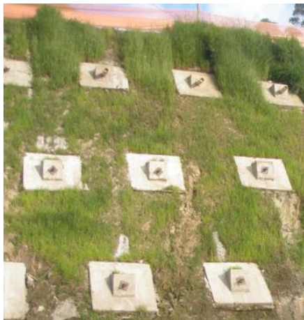
a) Support surfaces with individual concrete blocks.
