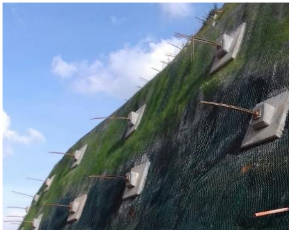
c) Individual concrete blocks with single twist mesh.
