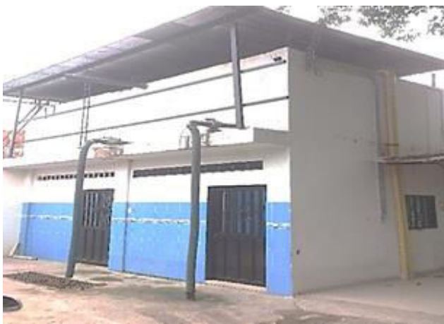
Figure-1. Physical plant, storage tanks.
