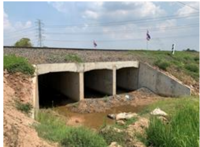
(b) Box culvert
