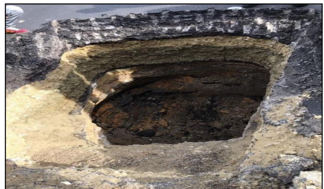
Figure-2. Excavation work to observe cavity beneath the pavement surface.
