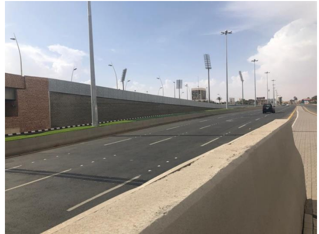
Figure-Error! No text of specified style in document.. Constructed MSEW at a highway, Hail Saudi Arabia.
