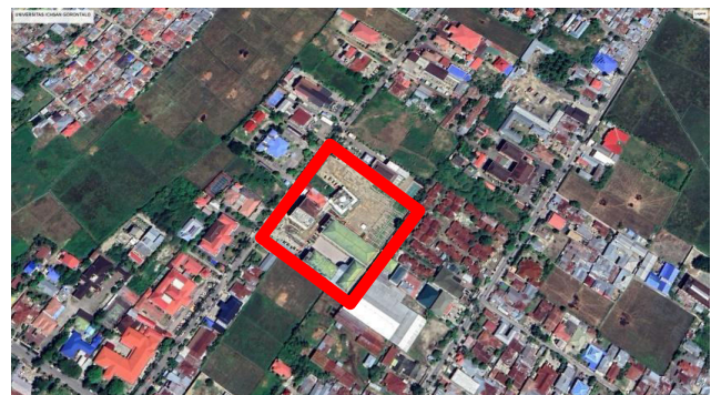
Figure-1. UNISAN Gorontalo building layout.
