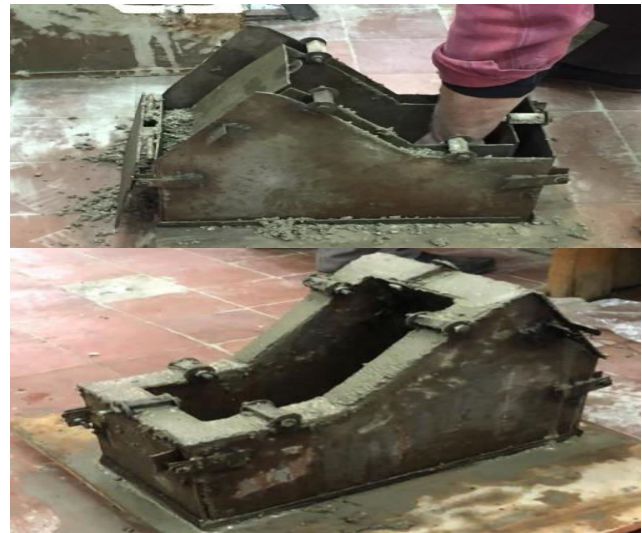
Figure-9(a) and (b). Casting the ventilation block.
