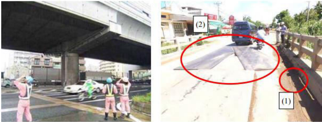
Figure-7. The routine inspection [75]
