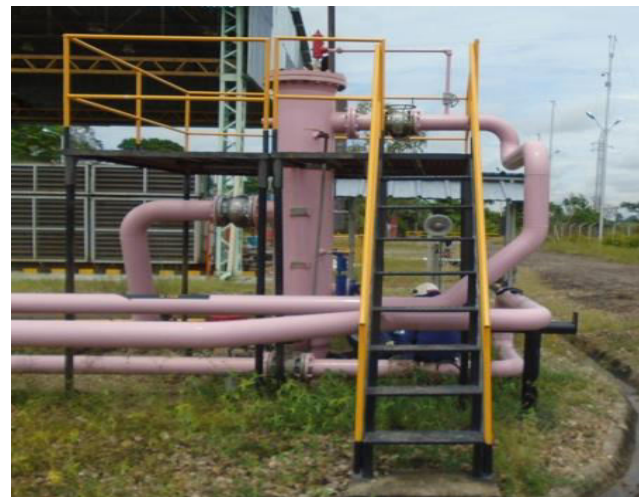
Figure-1. Vertical two-phase separator inspected.
