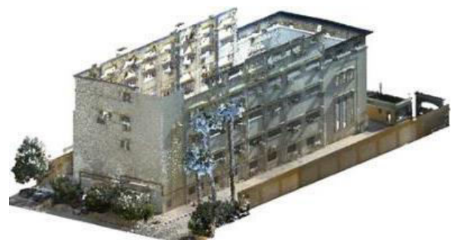
Figure-6. The 3D Laser Scanner Survey 3D Point Cloud Model Studying Building.
