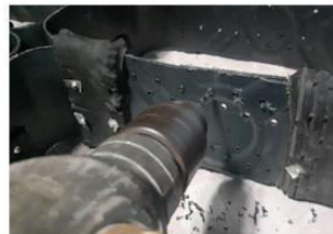
c) drilling of drainage holes
