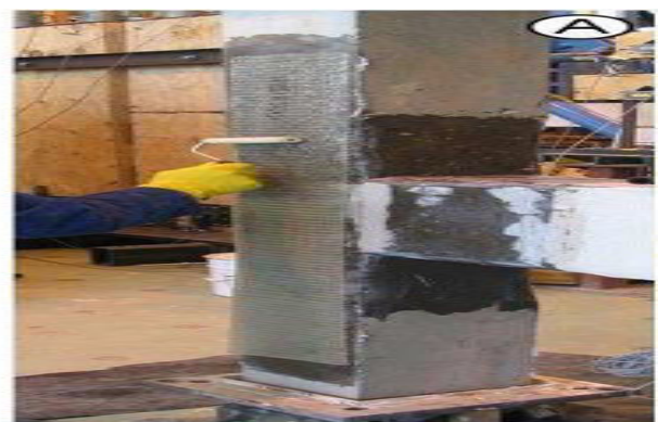
Figure-3.1. Vertical FRP layer application on column.
