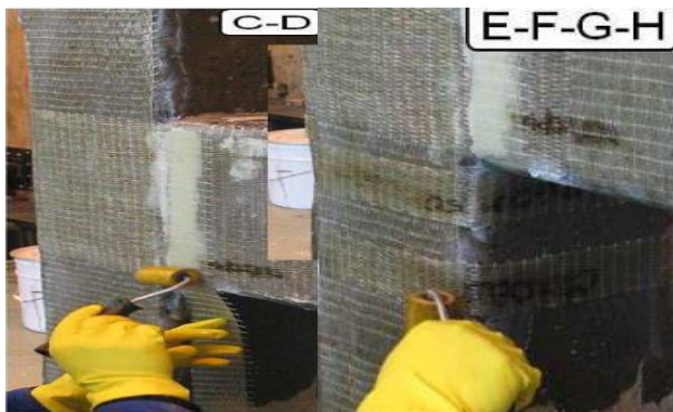
Figure-3.3. The additional smaller strips were also used to provide better anchorage to the main FRP laminates in the beam and column.
