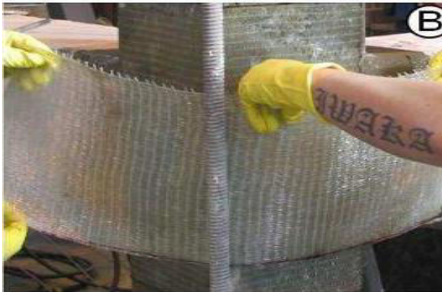
Figure-3.2. Application of U-shape horizontal laminate wrapped around the exterior column at the joint level.
